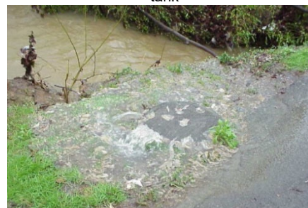
Wastewater overflowing down a busy street
